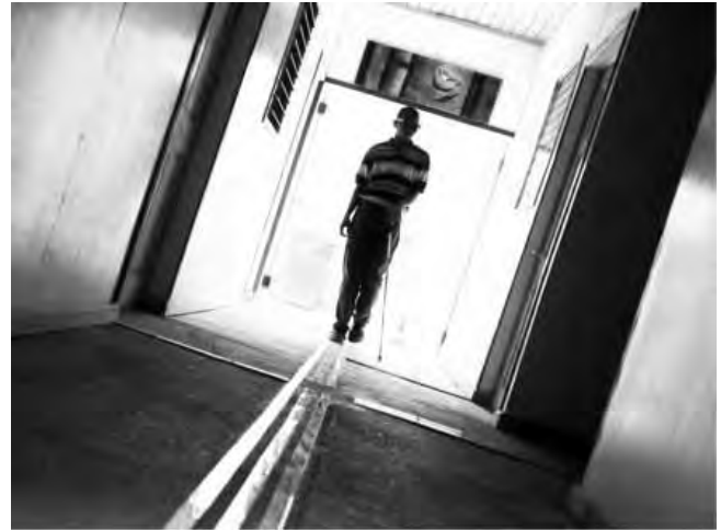
Tactile guideway in a public building in Haiti credits: CBM/ Frédéric Dupoux
