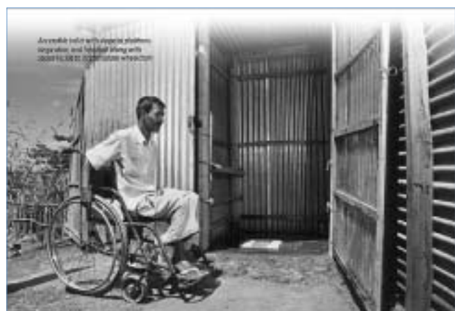
Accessible toilet with slope to platform, large door, and handrail along with space inside to accommodate wheelchair
